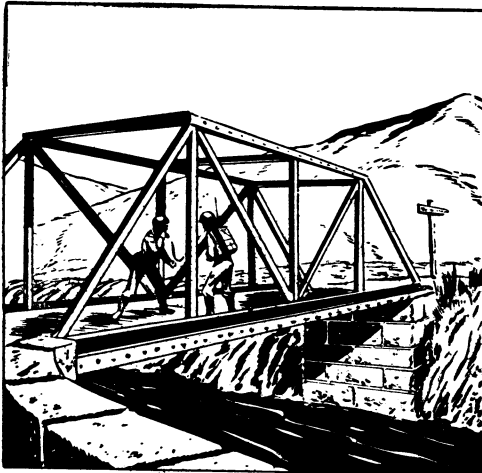
OVERHEAD STEEL BRIDGES
